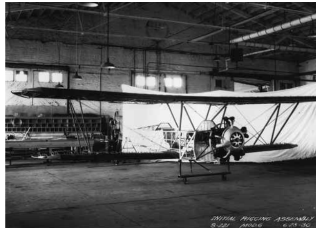
Initial rigging assembly
